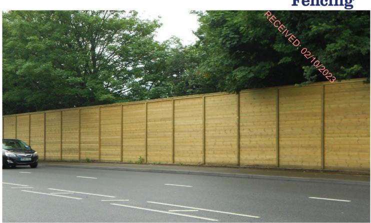
The Jakoustic® reflective barrier reflects the noise away using heavy section planed timber boards with a special profile that has been carefully developed. Boards are constructed in such a way that eliminates gaps that sound can easily travel through. Up to 28 dB\* in noise reduction.
